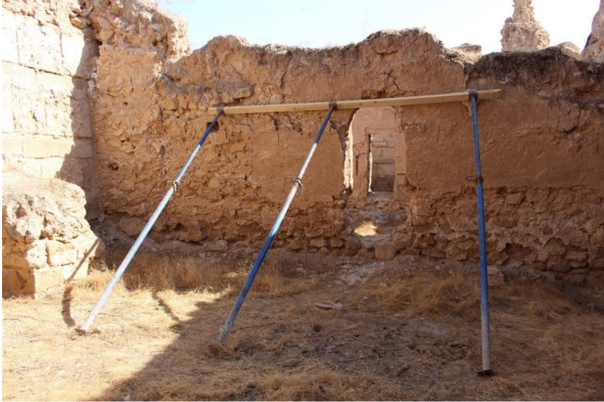
Fig. 67: The later wall supported by scaffolding pipes.
