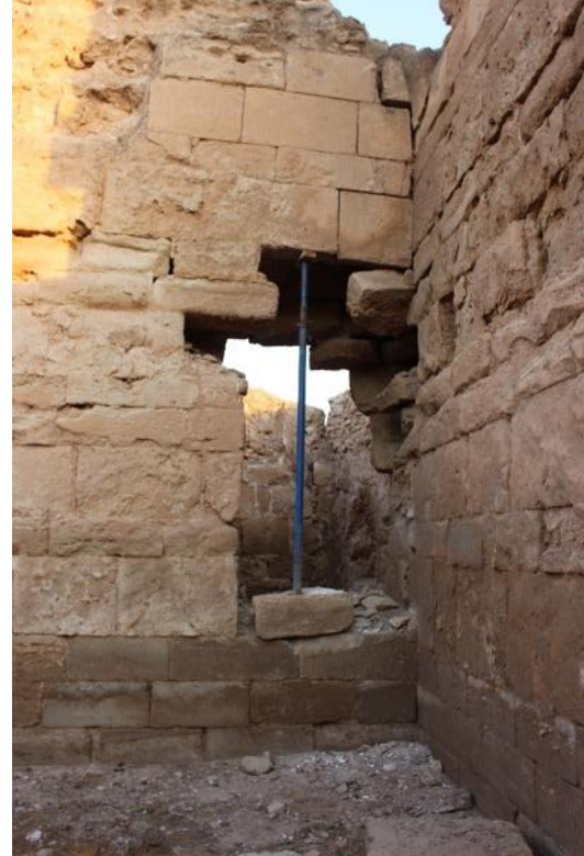
Fig. 64- 66: Shoring of the unsafe lintels.
