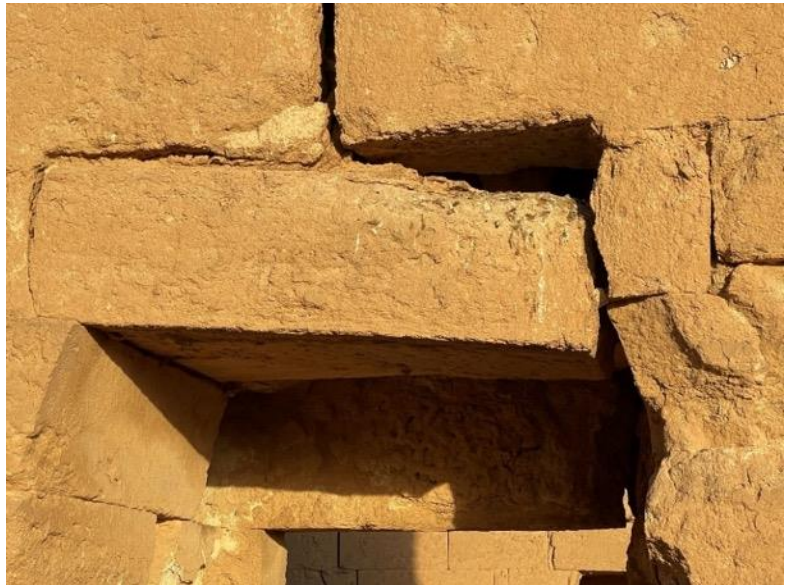
Figs. 56- 59: Crumbling lintel before and after the emergency intervention.
