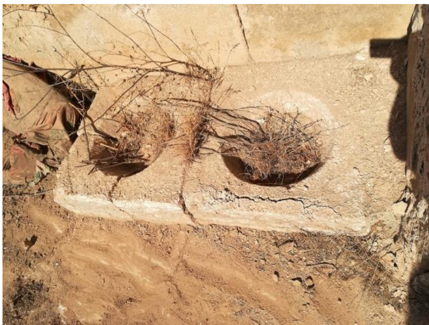
Fig. 61: Detail of two hemispherical cups with grass and bushes sinking roots directly into the decayed gypsum features.
