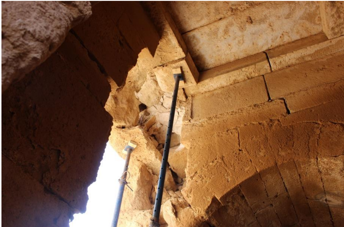
Fig. 64- 66: Shoring of the unsafe lintels.
