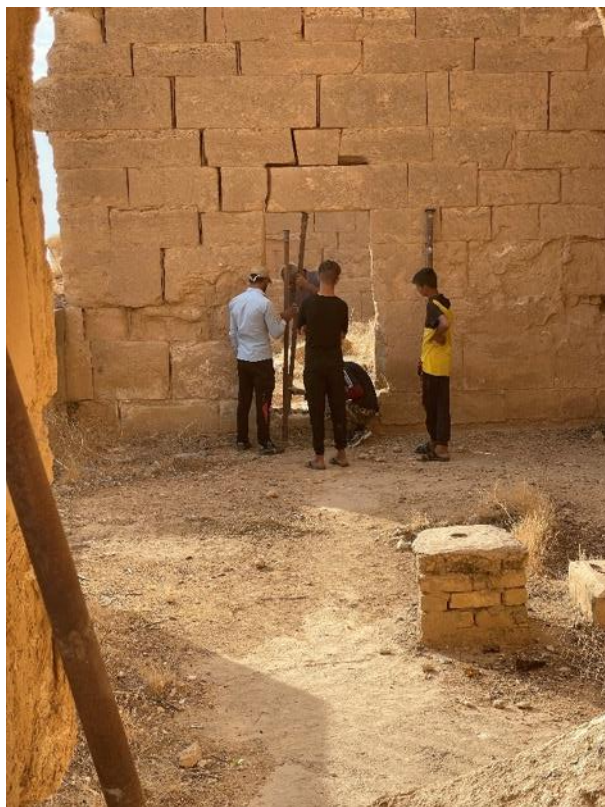
Figs. 56- 59: Crumbling lintel before and after the emergency intervention.
