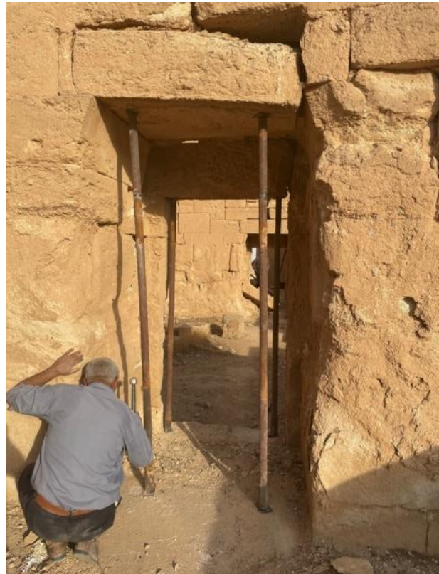
Figs. 56- 59: Crumbling lintel before and after the emergency intervention.
