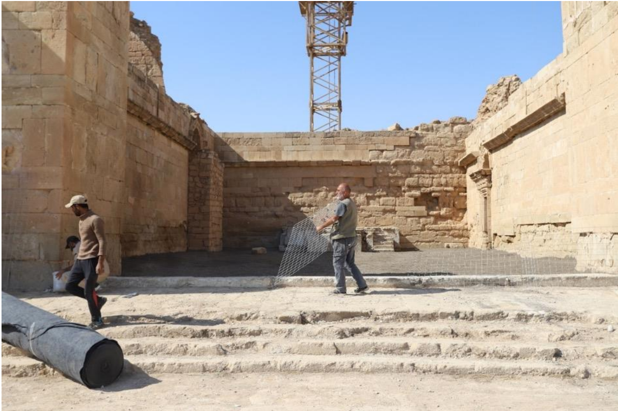
Fig. 43: Temple of Allat, central iwan with the entrance sealed with removable light iron frames and nets.
