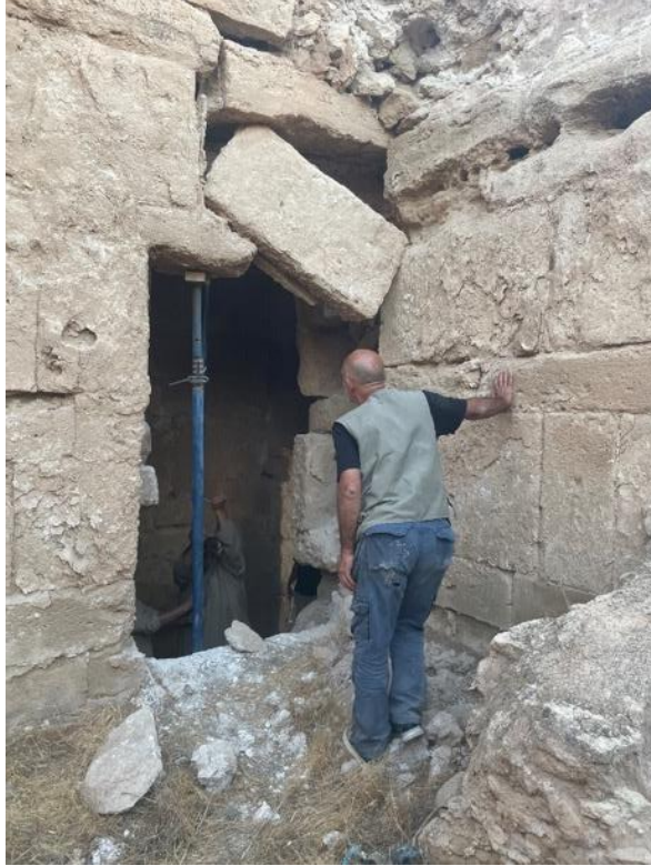
Fig. 64- 66: Shoring of the unsafe lintels.
